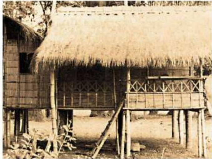
Traditional Kedayan home with grass-thatch roof, walls of tree bark, and verandah wall of split bamboo
